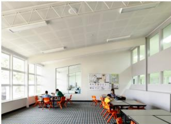
Classroom Ceilings: Raking ceilings to the top floor of the building allow for high level louvres to increase natural light and ventilation
